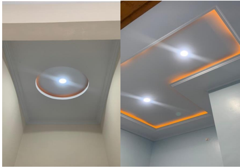
Gambar 3. Hasil finishing plafon gypsum
